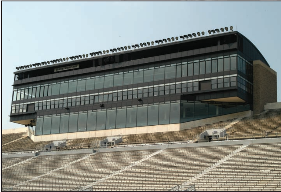
FIGURE 1. The thick concrete floor might have precluded other typical alternatives. The VRF installation avoided the need to cut through it.
