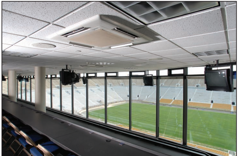
FIGURE 2. A constant air wash keeps the temperature constant in the glass-walled press box.
